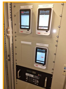
Control panel with flow computers
