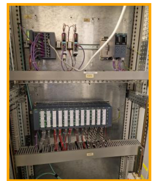
Control panel with flow computers
