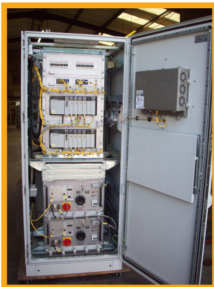
Bacchus MCS being built
