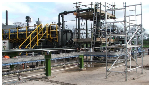
General view of a wellhead pad
