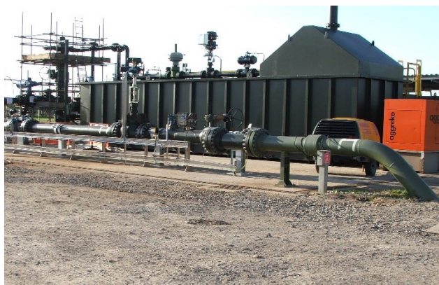
Photo of the first wellhead pad being tested
